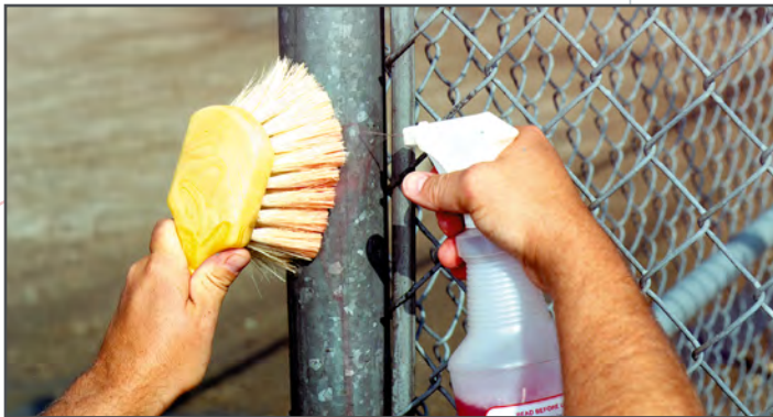
Cleaning galvanized steel
